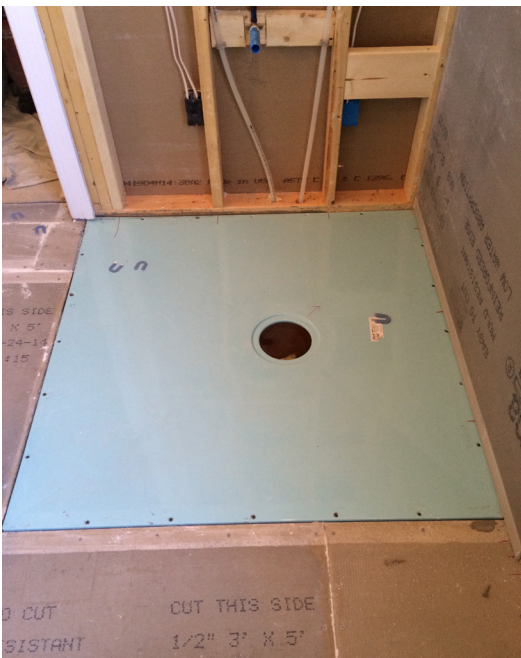
Classic shower base installed on joists.
